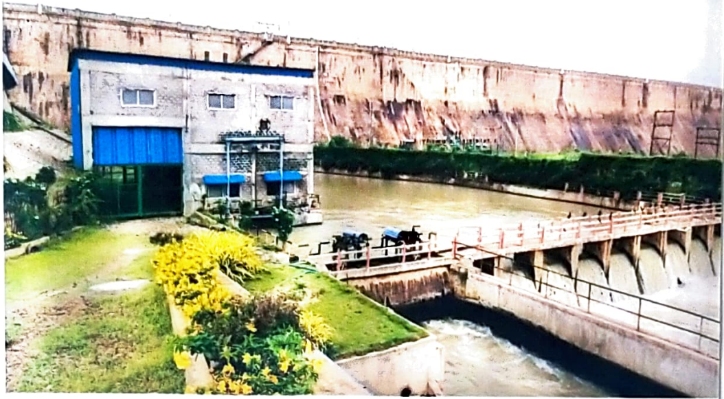
GENERATION OF POWER AT T.B. PROJECT.
