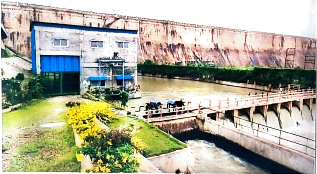
GENERATION OF POWER AT T.B. PROJECT.
