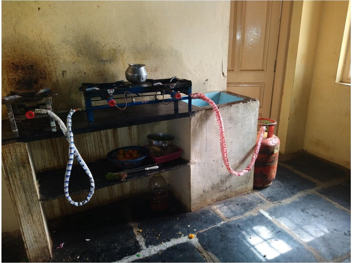
Figure 24 - Placement of LPG cylinders in wrong location.
