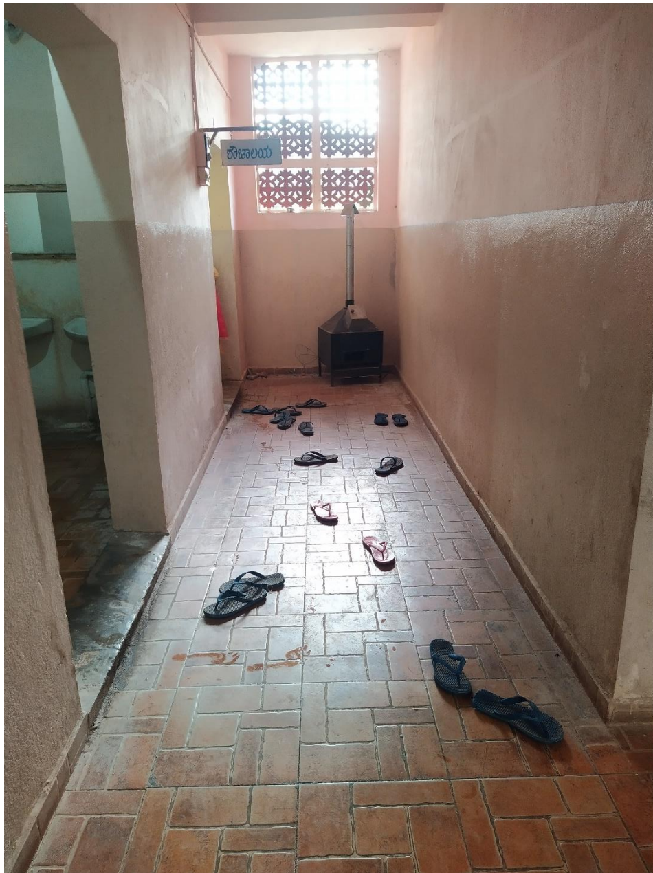
Figure 11 - Sanitary pad dispenser and incenerator.
